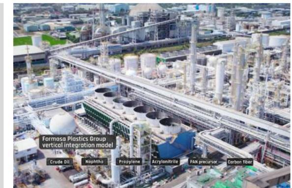
TAIRYFIL is fully vertically integrated from precursor to carbon fiber.
